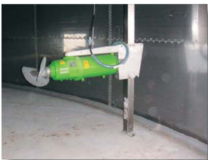
Proven submersible motor mixers for biogas fermenter vessels in a special pressure encapsulation for highest level requirements and durability
